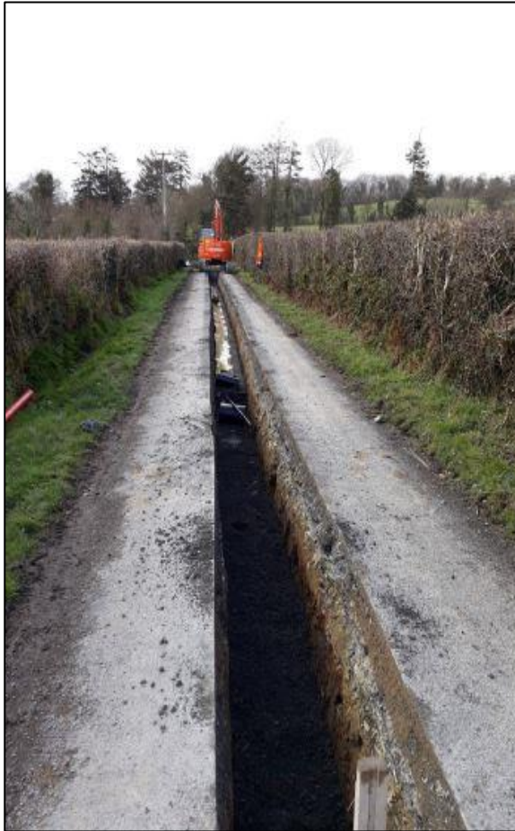
Figure 1 – Typical Trench Construction within roads
